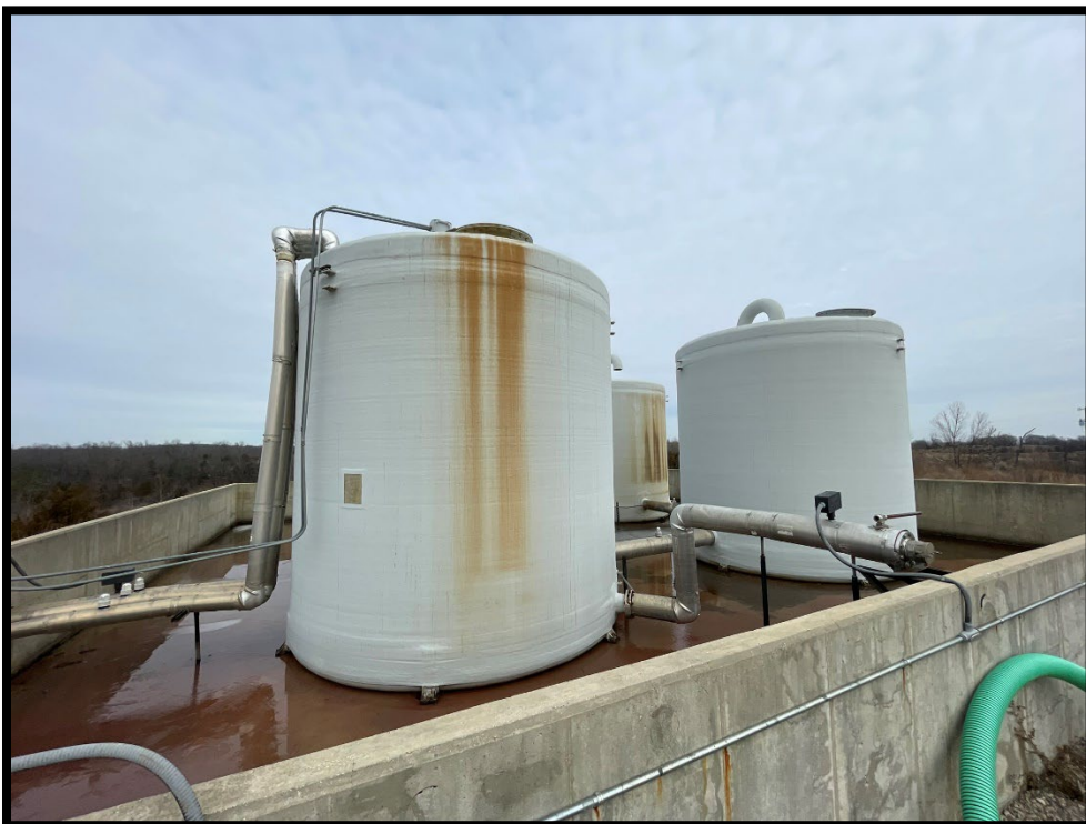
Photograph 2: View of minimal stormwater in leachate tank containment.
