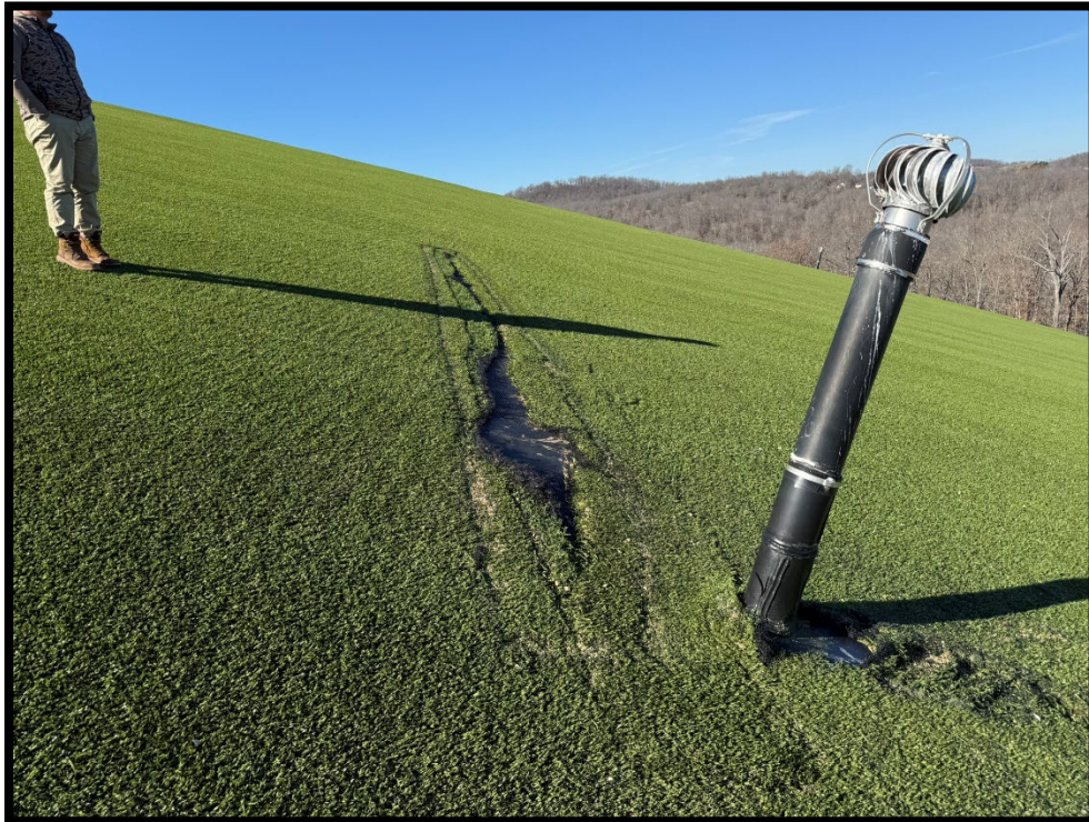
Photograph 3: View of DCT-1 on north side of Area 1-2, at 36.46181, -92.45045.
